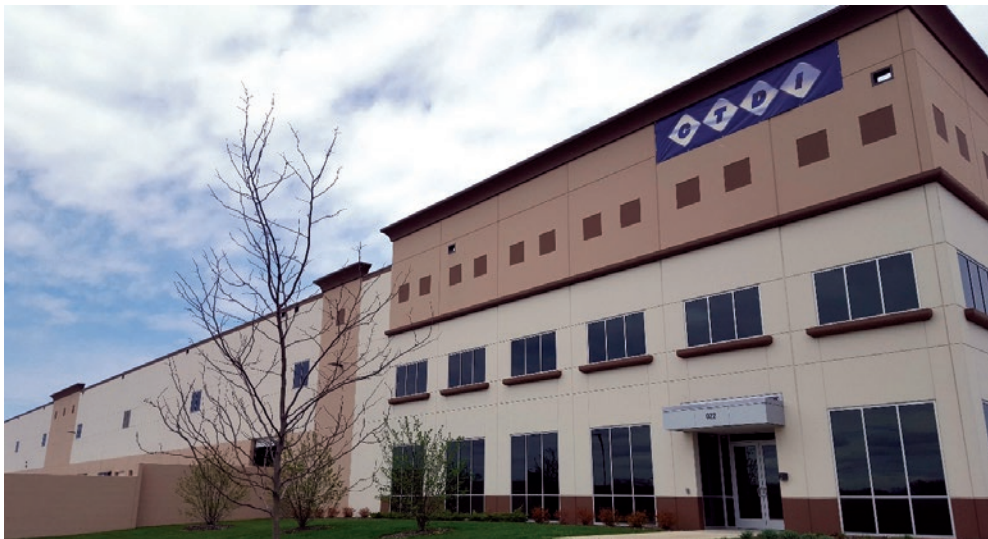
Communications Test Design Inc.'s new facility in Kenosha County is expected to create 150 jobs over the next three years.
