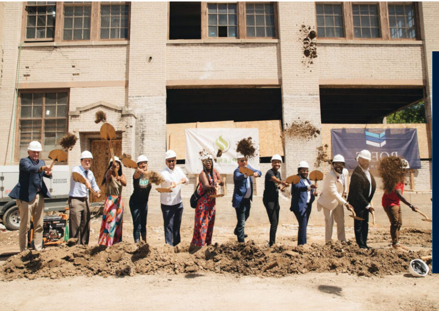
The Community within the Corridor project—which will provide 197 affordable housing apartments, a community center with child care, a food hall, a laundromat, resources for STEAM education and 25,000 square feet of recreation space—broke ground in June 2021.
