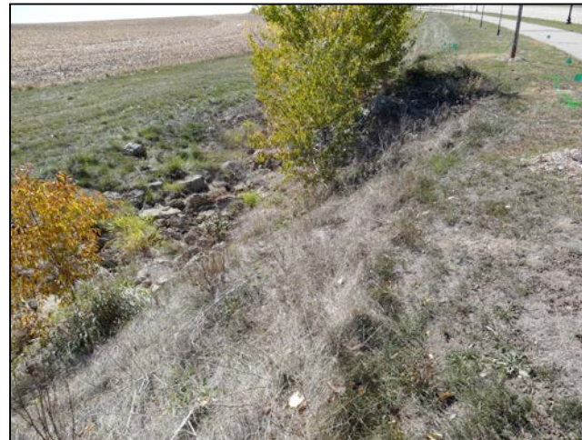
View of large culvert from roadside
