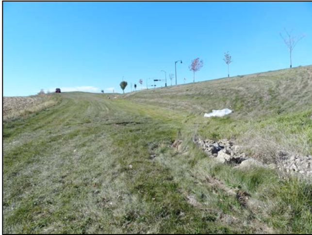
Riprap below small culvert – right side of photo
