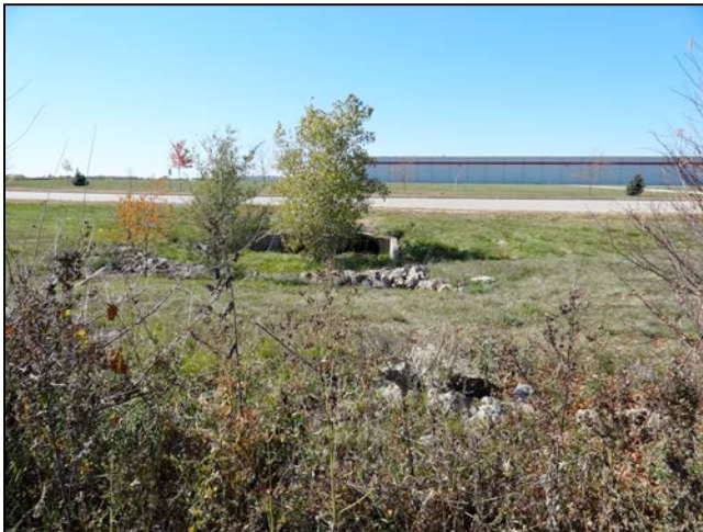
View of culverts under Gateway Blvd near data points 11 and 12, facing west
