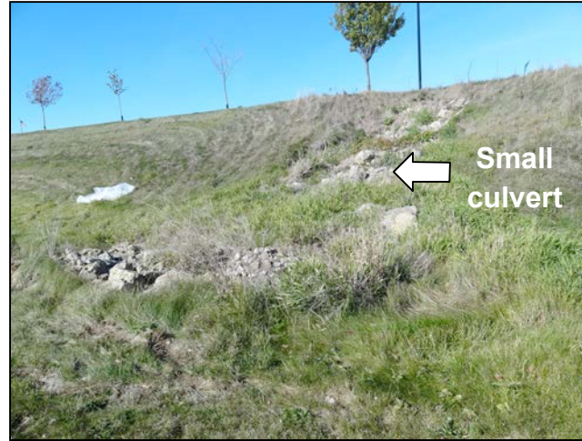
View of small culvert that drains Gateway Blvd
