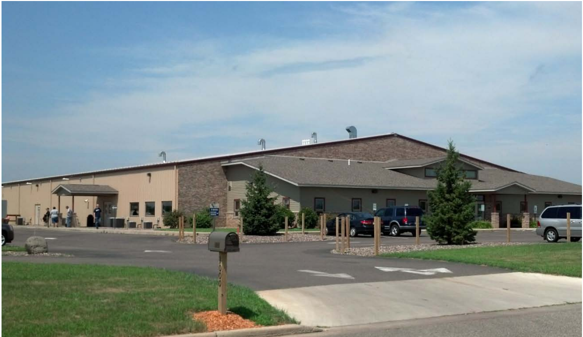
Photo 3 Chippewa Rivers Industries located on the adjacent property in the southwestern portion of the subject property.
