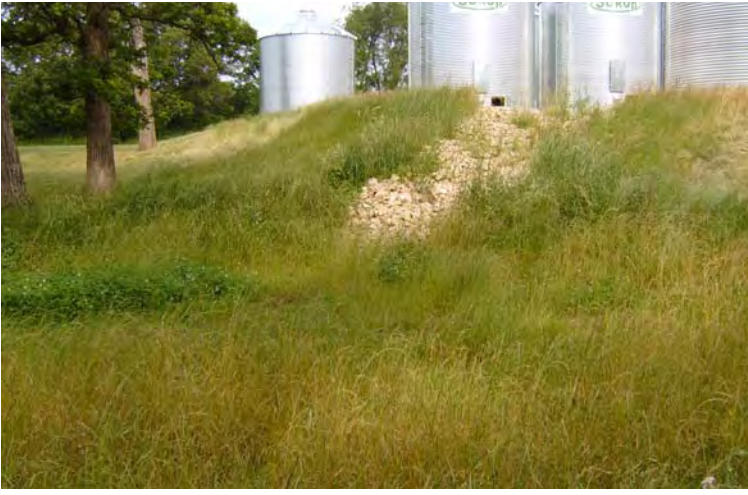
Small upland drainage from grain bins near W edge of delineated W-1 N boundary; Facing NW.
